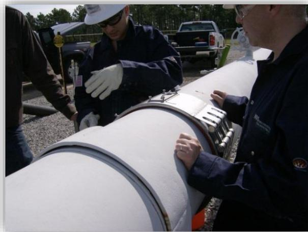
AE can be used for monitoring the ‘acoustic activity’ generated while hitting the pipe both accidental (digger hitting pipe) and intentional (theft attempt). Third-party interference are equipped with appropriate alarms that are sent to the asset owner or pipeline operator.
