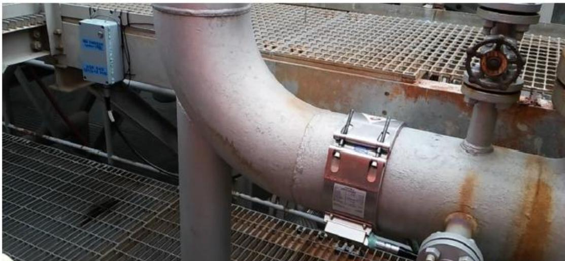
**Figure 4** Example of SpotOn® U installed at pipe in Aromatic unit
