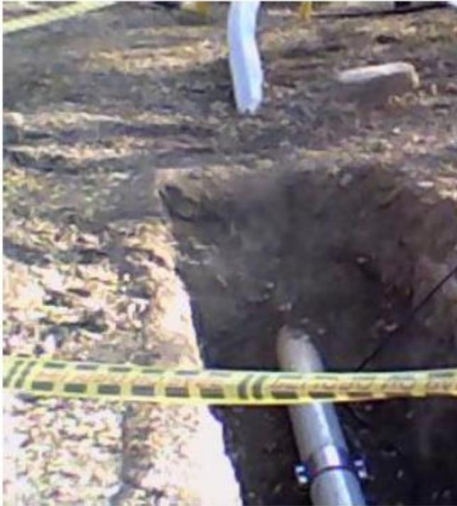
**Figure 8** SpotOn® U example installation at E&P facility. The sensor was buried and the comms unit was placed above ground
